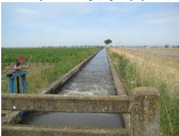
Figure n°1. Irrigation de surface.
