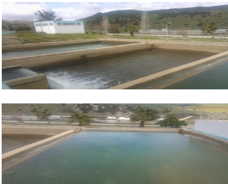
Figure 09: Bassins de filtration
