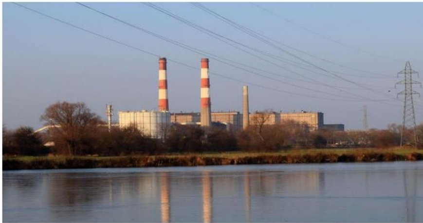
Figure 1.4: Photograph of a thermal power plant [10]
