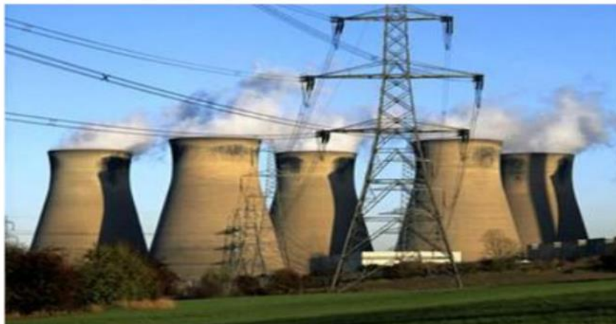
Figure 1.7: Photograph of a nuclear power plant in France.[10]
